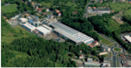
AGC Brevka plant in the Czech Republic
