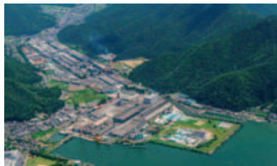
NSG Group's plant in Maizuru
