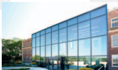
Hugel Welcome Center in Markle Hall on the campus of Lafayette College in Easton, PA, the first project in the U.S. to feature VacuMax™ VIG - Photography: Jim Cunningham
