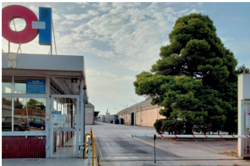
O-I plant in Marsala
